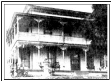
The former S. D. Freeman Sanitarium 110 E. King St. is now a rental unit.
